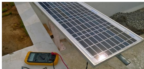
Fig 6.1.a: Solar panel output checking with multimeter
